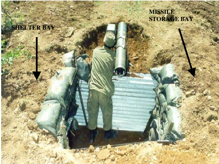
Figure 2-23: Eryx Trench—Stage 2, Rear View
